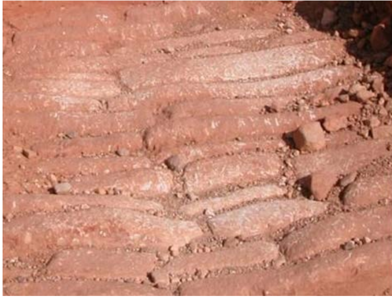
Photo 11.13 - Rip Rap Armoring
