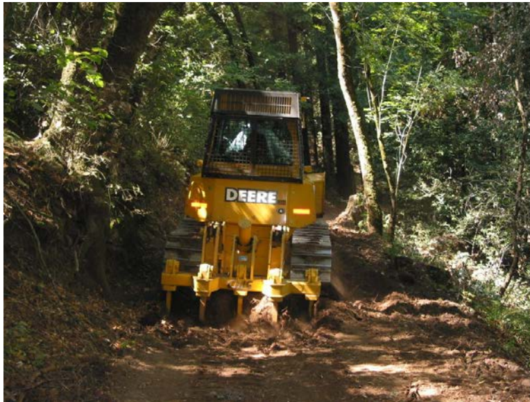
Photo 11.17 - Dozer Ripping Road Bed
