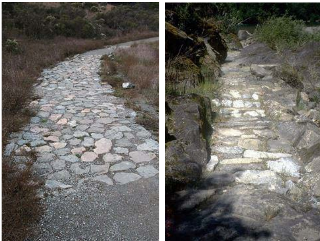
Photo 11.12 - Applications of Stone Pitching
