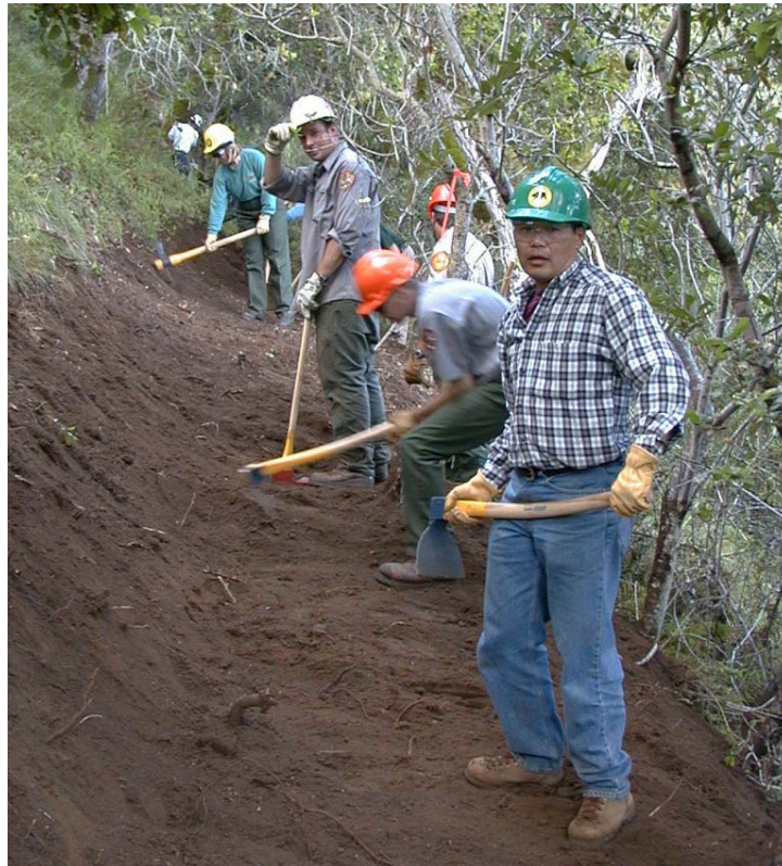
Photo 11.4 - Stagger Line to Reduce Worker Movement
