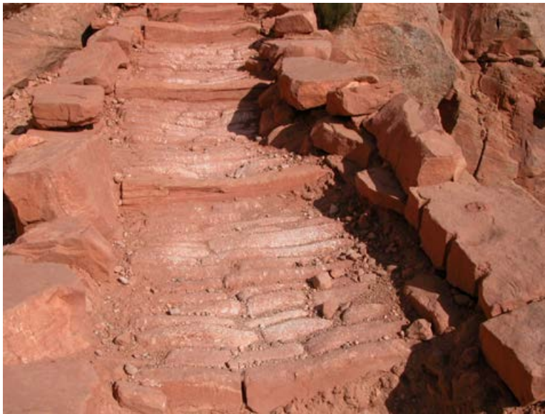
Photo 11.14 - Rip Rap Used with Rock Framed Steps
