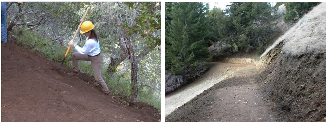
Photo 11.7 - Dispersing Sidecast Soils
