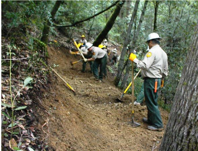
Photo 11.3 - Workers Sidecasting Soil
