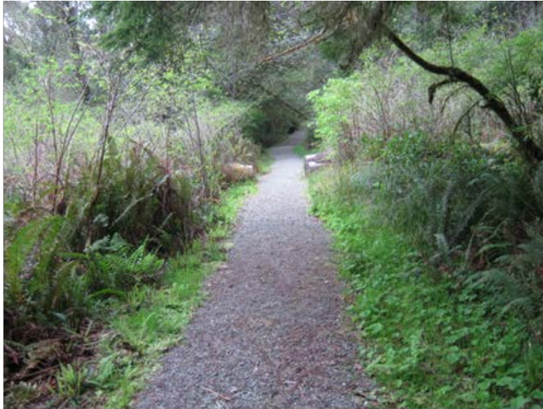
Photo 11.11 - Aggregate Surface
