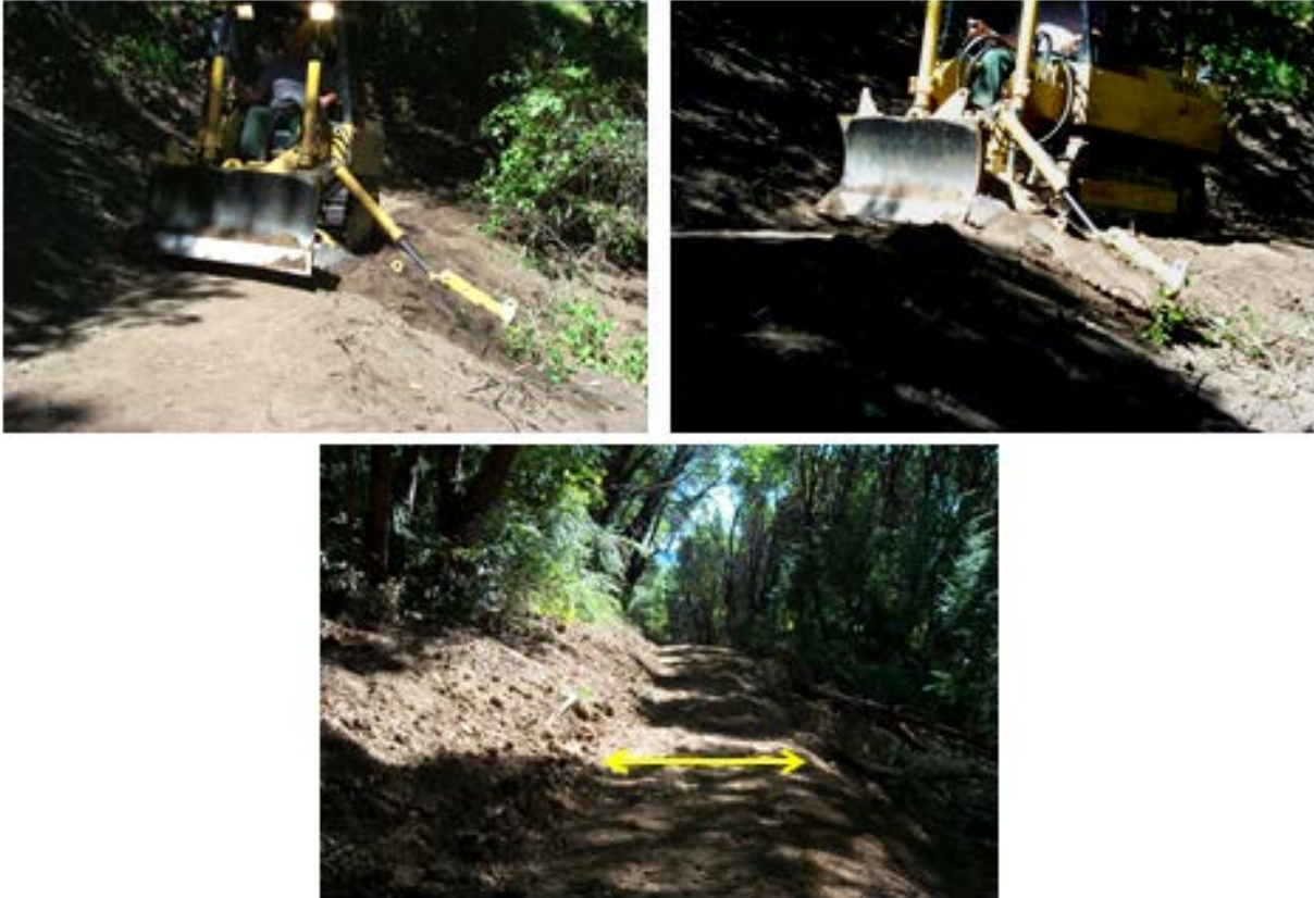
Photo 11.19 - Small Dozer Trail Construction
