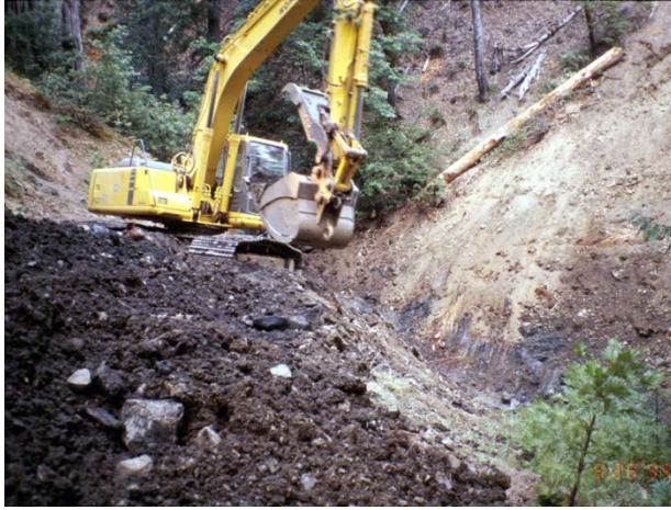
Photo 11.23 - Watercourse Crossing Removal During and After
