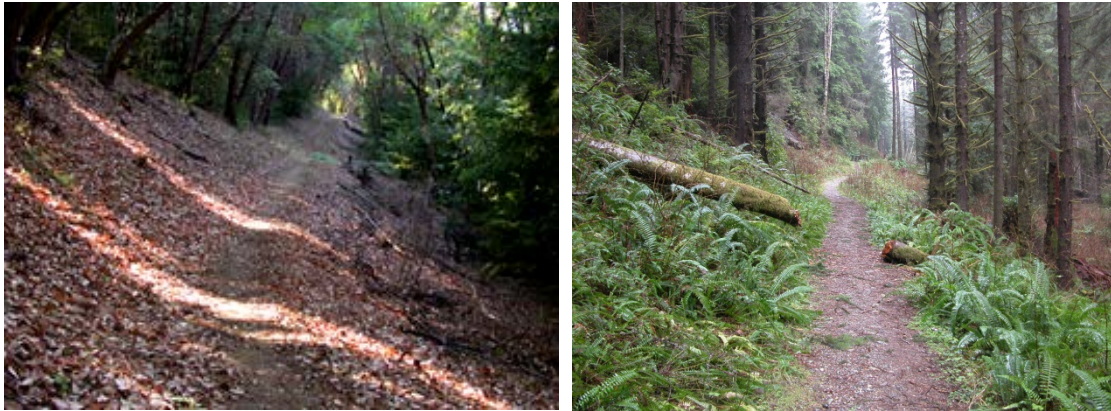
Photo 11.21 - Completed Road to Trail Conversions
