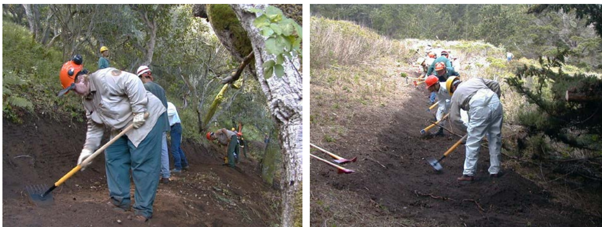
Photo 11.5 - Using McLeods for the Final Shaping
