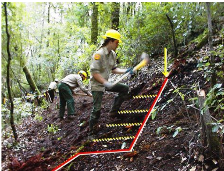
Photo 11.2 - Lead Worker Begins First Cut
