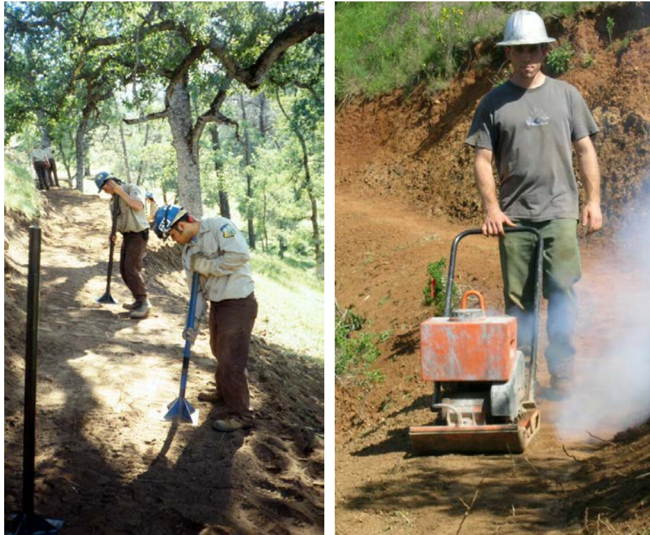
Photo 11.6 - Compacting the Trail Tread with Hand Tamper and Plate Compactor
