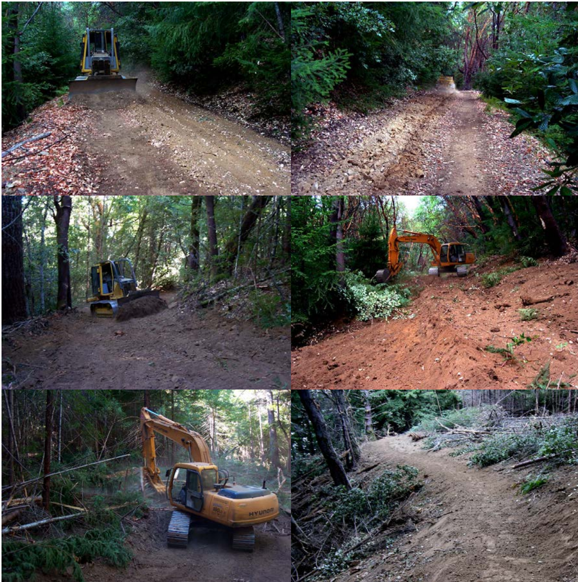
Photo 11.18 - Sequence of Heavy Equipment Trail Construction
