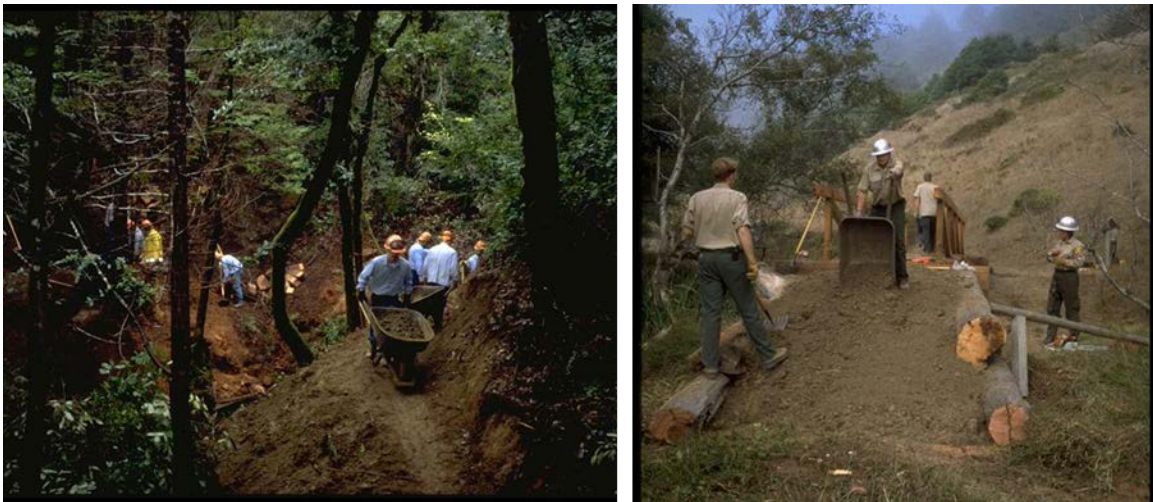
Photo 11.9 - Exporting Excavated Soil
