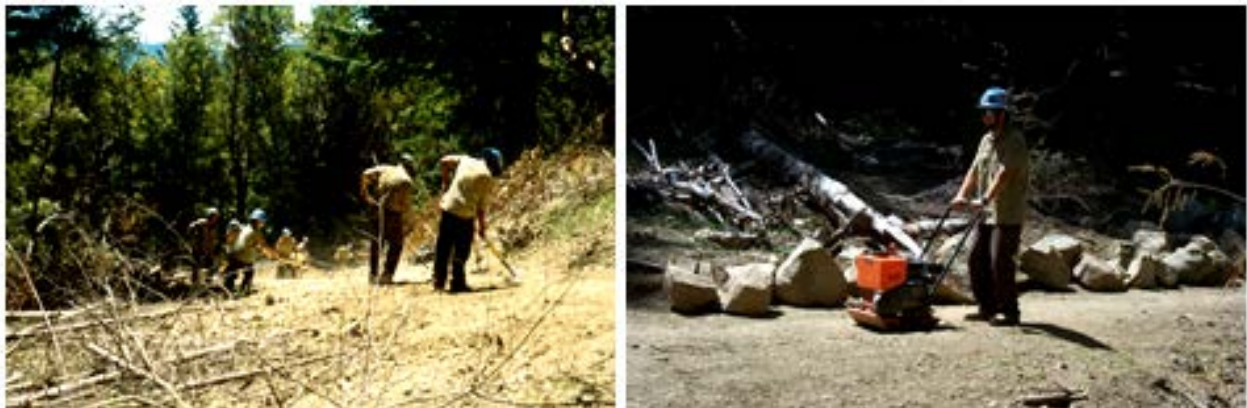
Photo 11.20 - Hand Crews Performing Final Trail Construction
