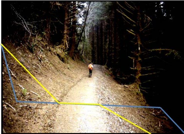
Photo 11.15 - Blue Line is Original Road Profile; Yellow Line is Native Bench
