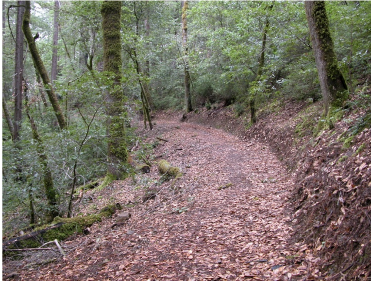
Photo 11.8 - Finished Trail Tread with an 8% Linear Grade and a 16% Outslope
